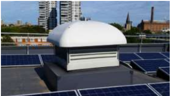
Supplier: Monodraught – X-Air Thermal Mixing Unit
