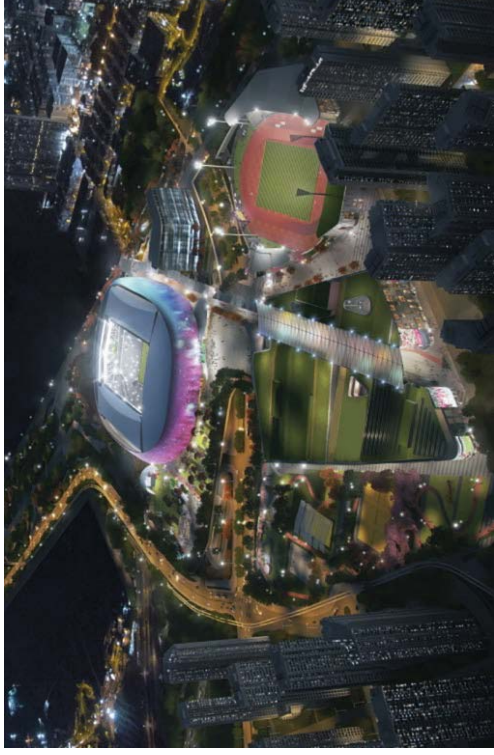
Overall View – Night-time
