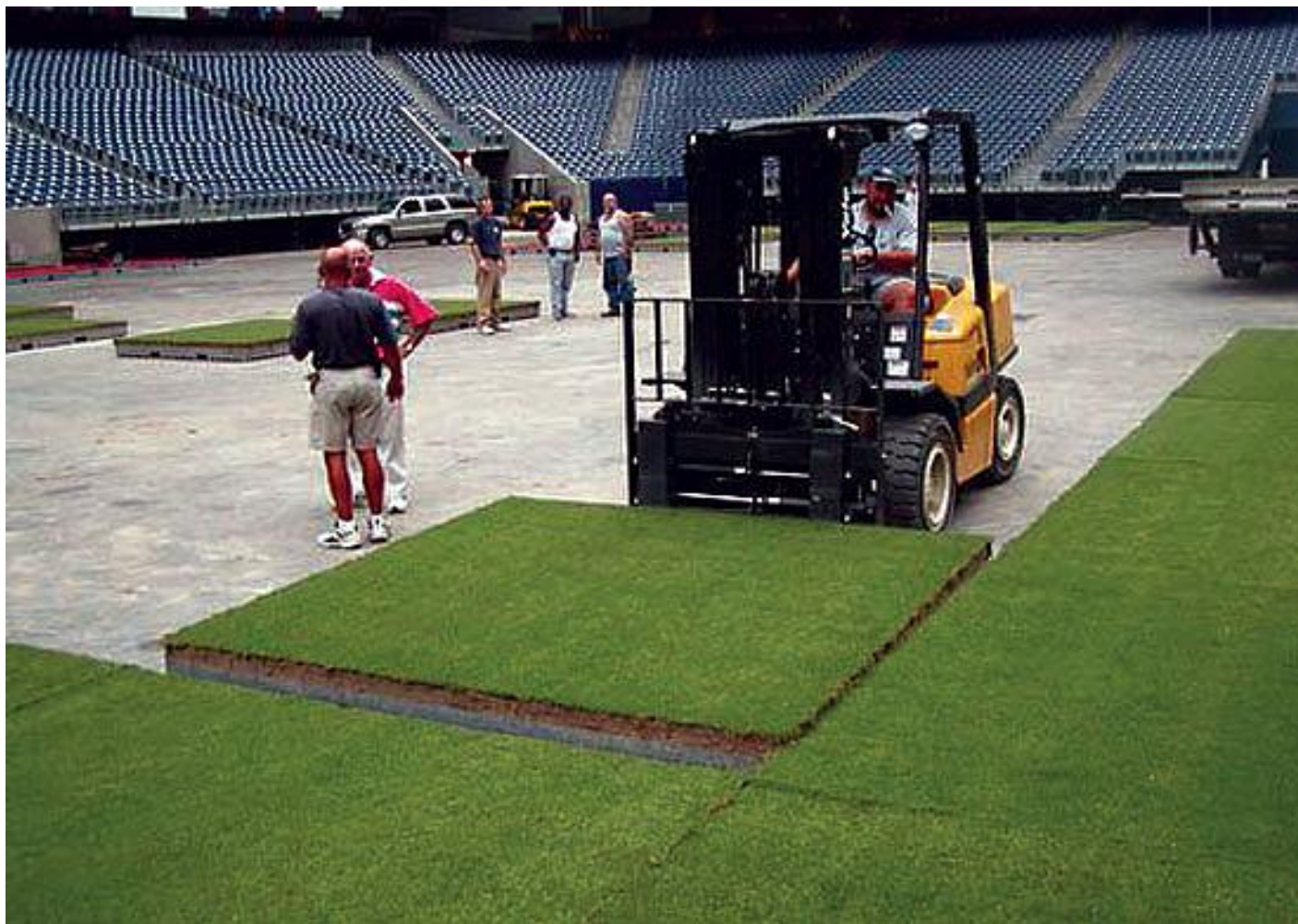
Palletized Turfing in Progress 塊裝草披鋪設中
