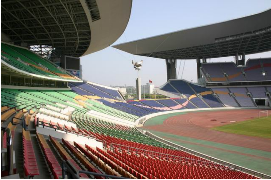
Guangdong Olympic Stadium
